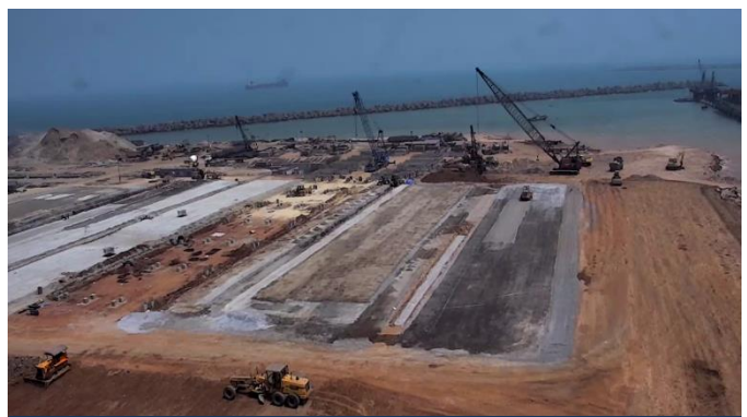
Yard reclamation work in progress
